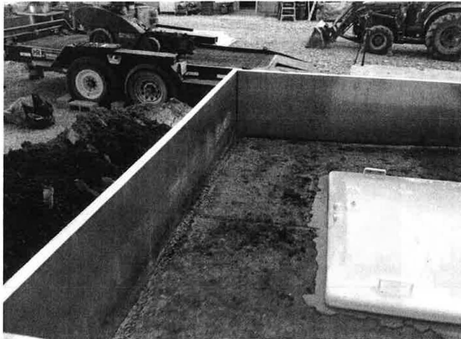
Figure 15 – Bentonite chips placed along the inside of the outer ring
