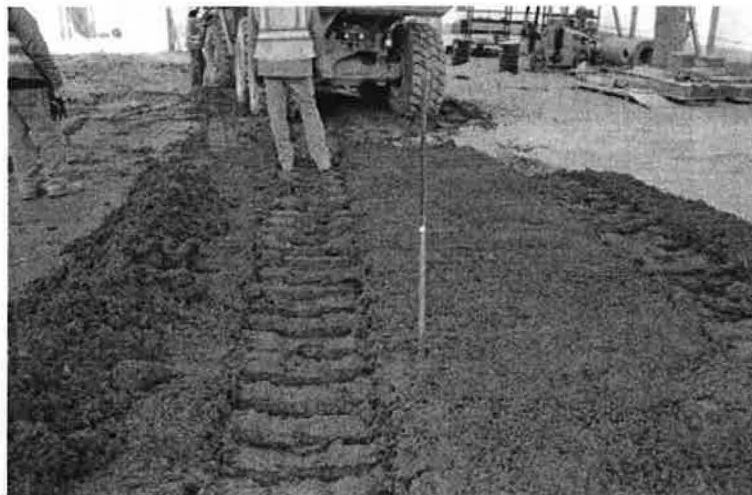
Figure 9 – North side lift 1, 12 inch loose
